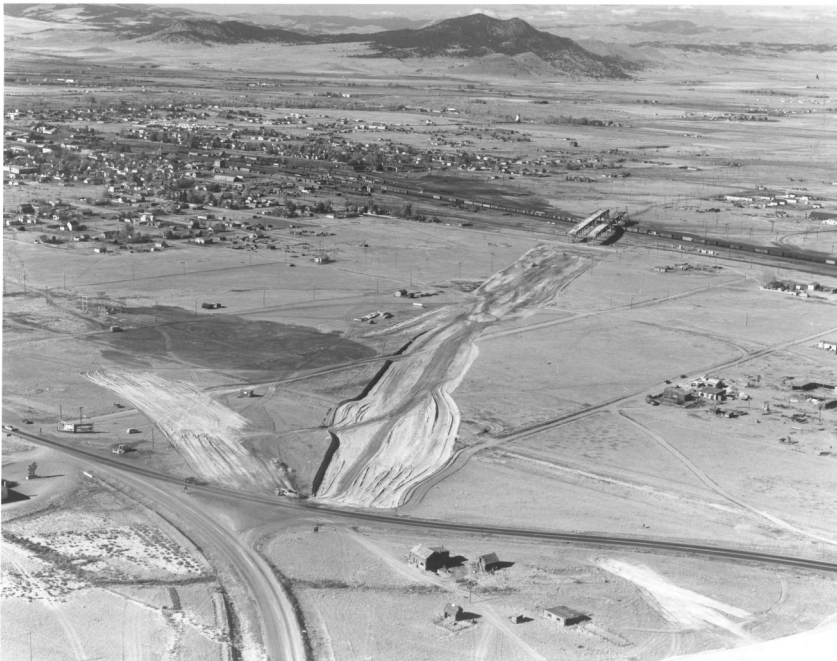
I-15 construction in Helena
